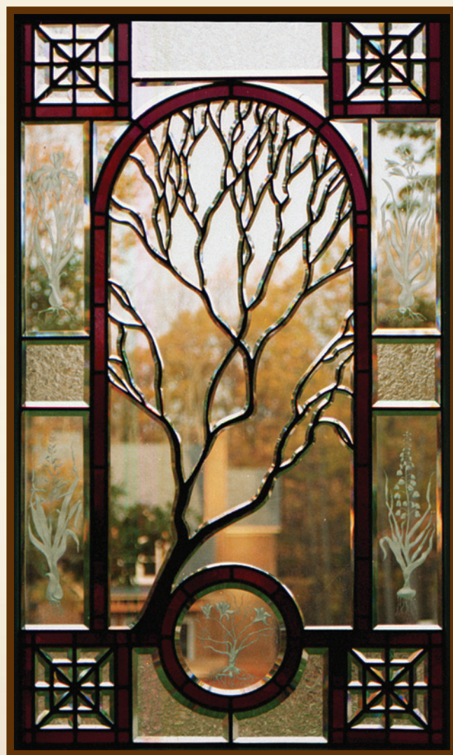
A solder sculpted and beveled residential window installation.
