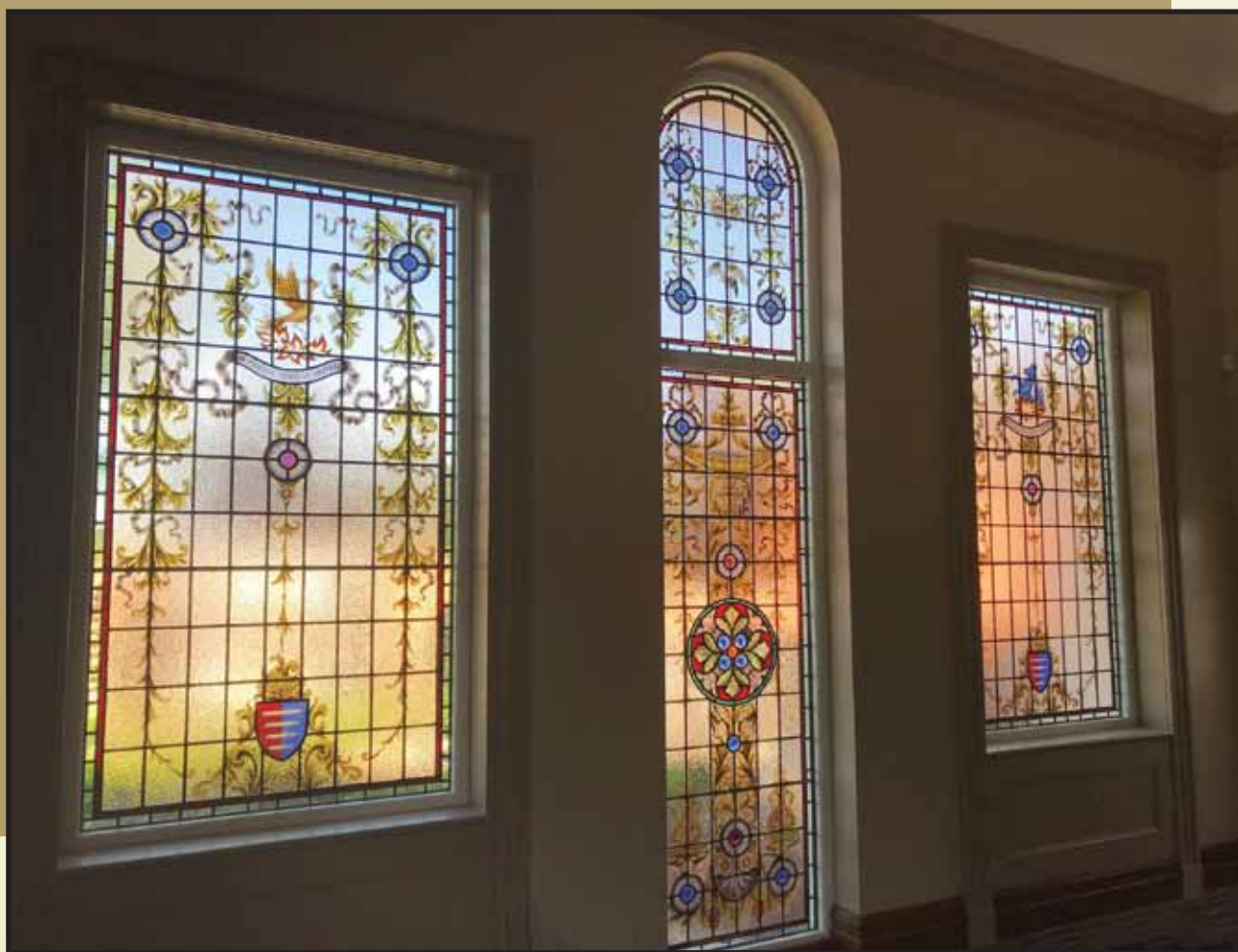
Juliet Forrest, Heraldry Windows, leaded windows created using painting, silver staining, and enameling, 130 cm x 240 cm (each window), 2019. Juliet designed and created the two rectangular windows flanking the central antique window, which had been relocated within the house due to extensive renovations. The brief was to match with the antique panel while also incorporating elements of the client's coat of arms. It was key to ensure impeccable matching across the glass, paint, stain, and enamels to ensure the new and the old sat well together.
