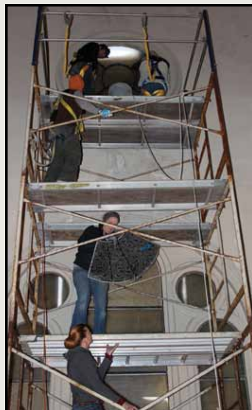
Removing the rose windows from St. Maurice
